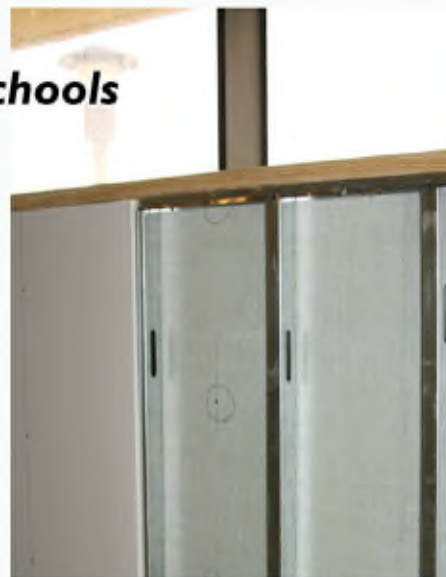
ArmorCore panels installed on stud wall for bullet resistance
