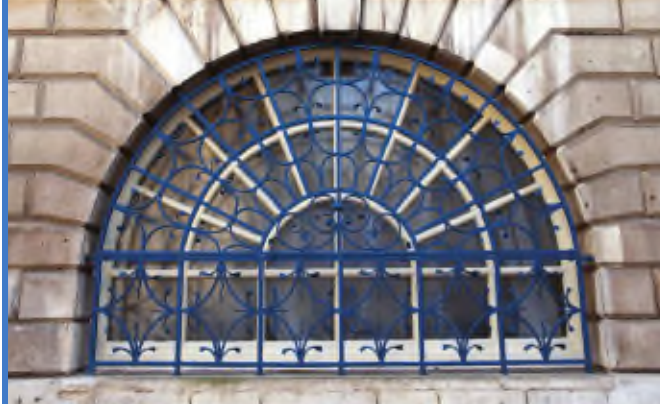
Figure 3: A security screen over an existing window reduces the potential for forced entry.
